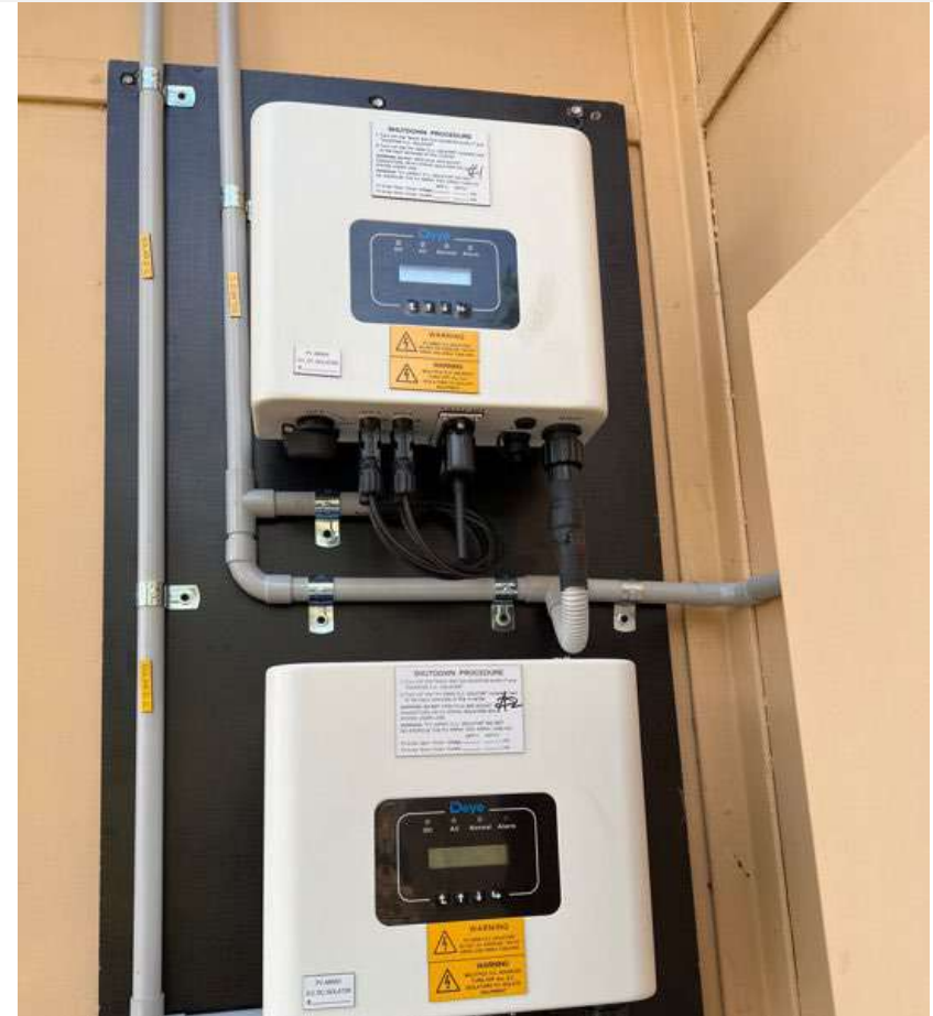
5KW PV Grid-tie Hybrid, VIC
