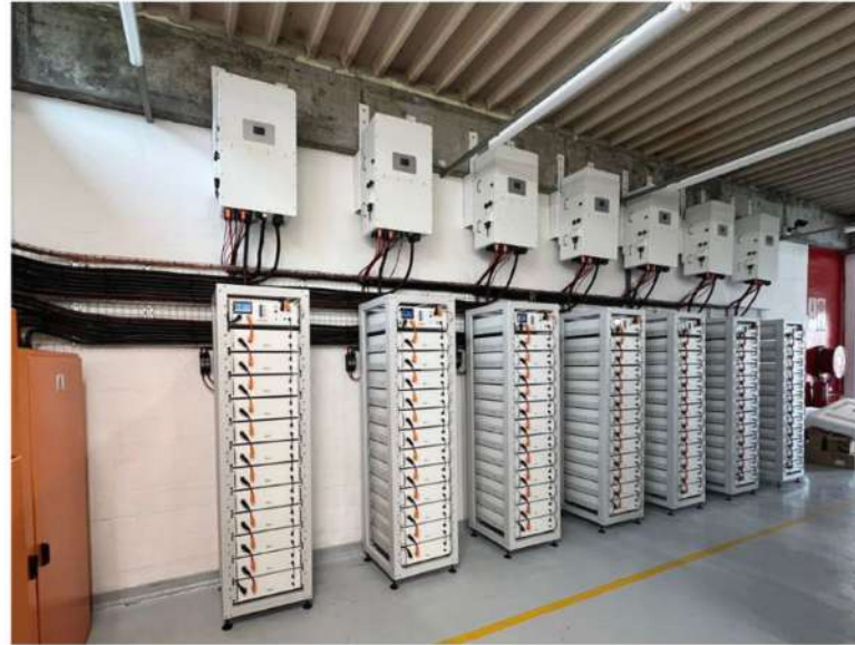
Inverter: SUN-50K-SG01HP3-EU-BM4*7(pcs) Battery: BOS-G
