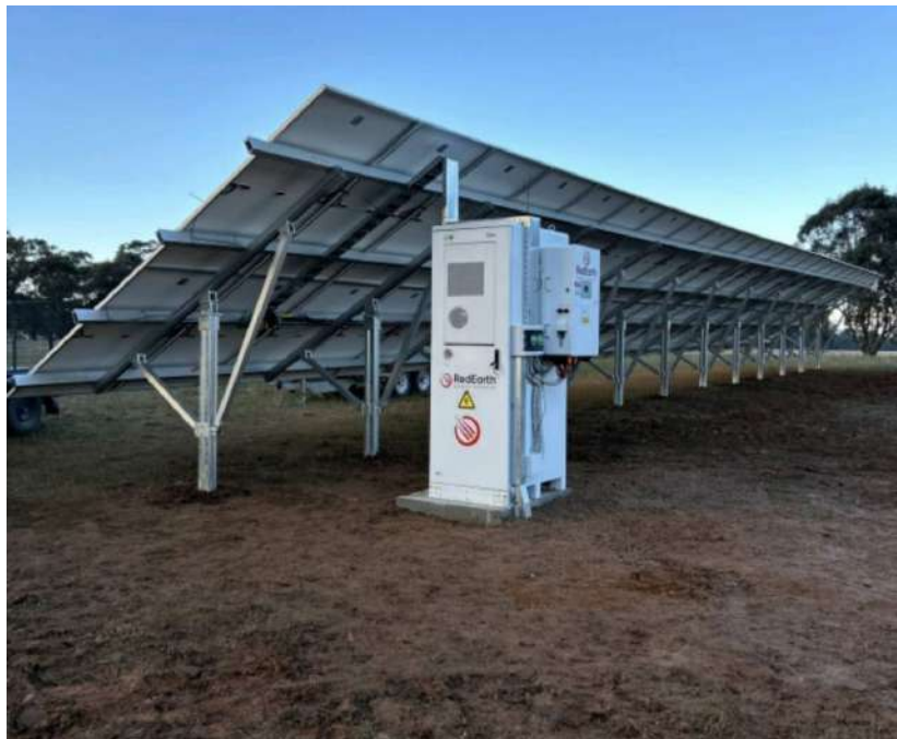
Deye 50kW/60kWh ESS in QLD Australia
