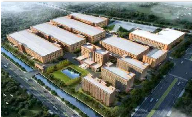
HaiYan Factory - Completion in 2025
